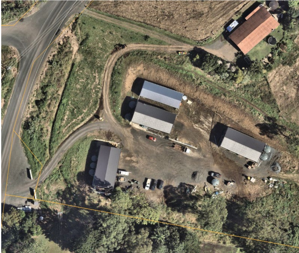
Figure 4.3 – View of existing access and available parking areas
